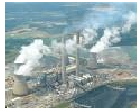
Georgia Power's Coal Burning Plant Bowen in Euharlee, Ga
